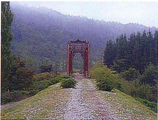
Disused railway bridge – Angol – Chile 📍 37° 49' 50.03" S, 72° 43' 21.61" SW Puente del ferrocarril en desuso – Angol – Chile 📍 37° 49' 50.03" S, 72° 43' 21.61" SW
