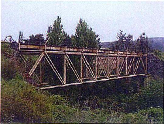
Disused railway bridge – Chile Puente del ferrocarril en desuso – Chile
